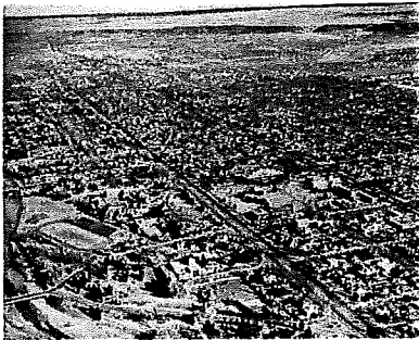
Aerial view of the campus looking north (photo c. 1940).
