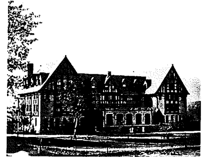
Bemis Hall, a women's residence hall, was built at the south end of Wood Avenue in 1908. Maurice B. Biscoe, New York, architect (photo c. 1920).
