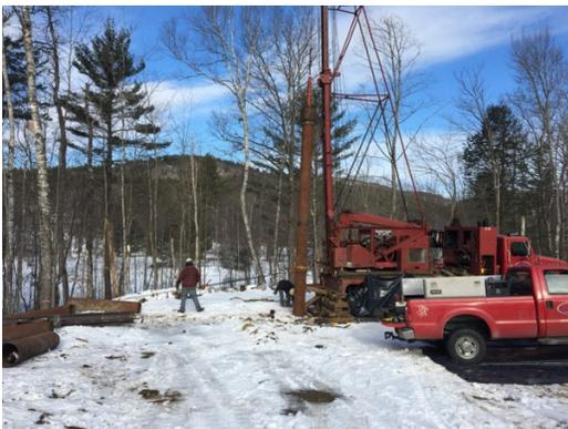
*Sometimes old technology is the way to go - drilling a spring water production well in an esker deposit in the western Maine mountains using a cable tool rig from the 1940's.*
