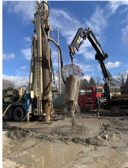
*Drilling a 24-inch water supply well on a military base in northern NJ with a dual-rotary rig.*
