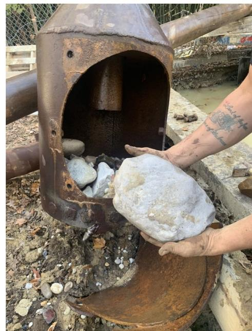
*Using unconventional tools to remove large cobbles from a well being drilled using flooded reverse rotary in the upper Potomac-Raritan-Magothy aquifer in southern NJ.*
